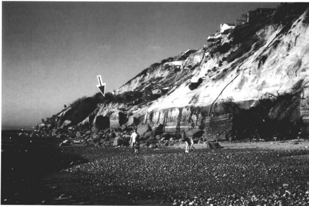
Figure 12. Recent blockfalls and translational landslide in sea-cliff, Leucadia, California. Blockfalls and landslide (arrow) utilized BPS at base of cliff as basal failure surface.
