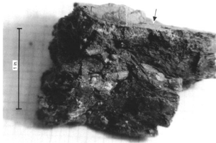
Figure 11. Gouge zone showing anastomosing shears and upper slip surface (arrow) of BPS in Border Patrol roadcut.
